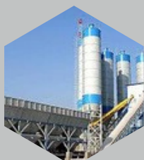
Ready Mix Plant
